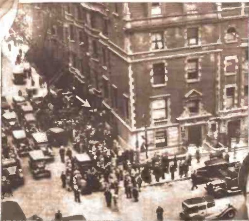
The building at 303 West 90th Street, where Crowley was cornered by a cordon of 800 policemen summoned by short wave radio calls
